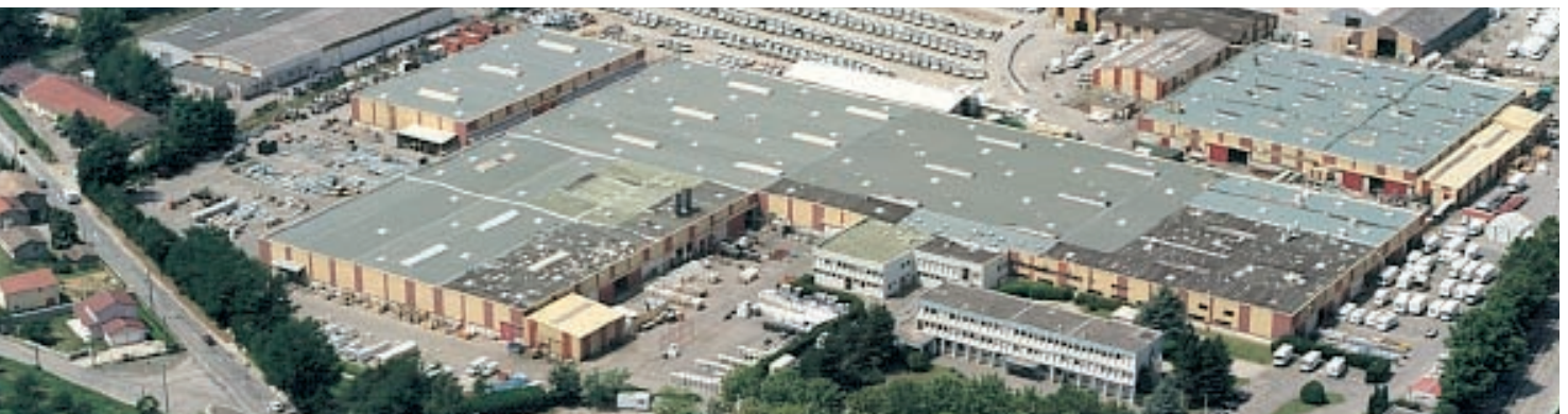
Aerial view of the leisure vehicles plant at Tournon-sur-Rhône (France)
